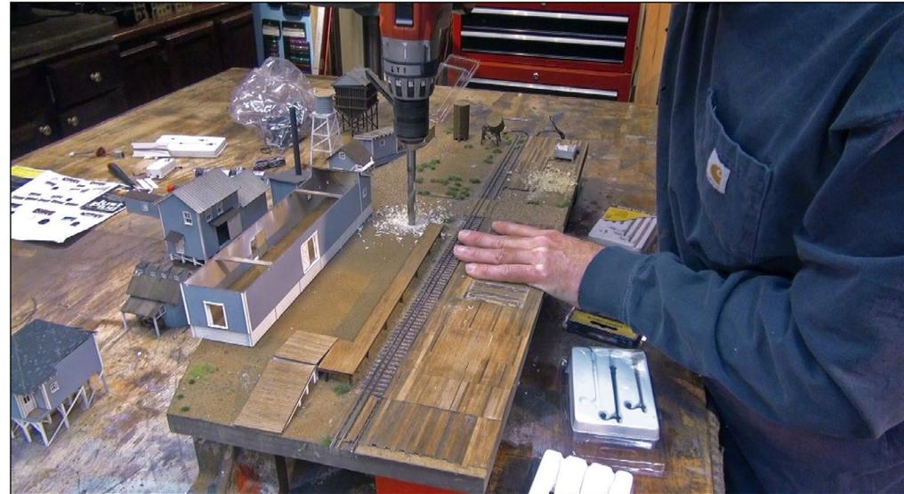
24.: Using a 3/32-inch bit, I drilled eight holes through the 3/4-inch plywood base to accept the lamps. I also drilled 1/2-inch holes in the scene to feed the wires up to the buildings.
