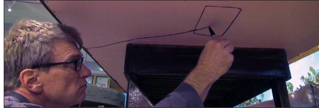
12. Underneath the layout, I used a Sharpie to draw a rectangle where the light hubs will be installed. I also drew a line from the auxiliary switch to the square where I will run the switch wires. Using a box knife, I cut a slot in the foam where the wire will run to the hubs. I used a screwdriver to press the wires into the slot, embedding them permanently in the foam.
