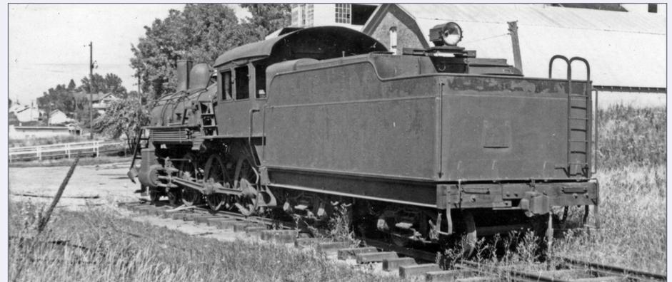
35. In temporary storage behind the Potlatch depot, we get a good view of Number 1's tender. Originally built with a coal bunker, it was converted to an oil bunker in 1912. During WWI, the engine was switched back to burn coal, and then re-converted to oil at the end of the conflict. Ivan Ergish photo, WI&M Ry. HPG collection
